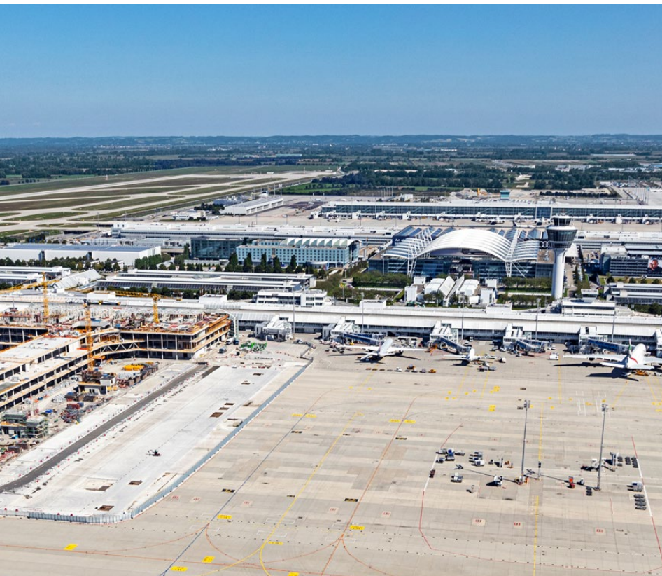
The structural work for the new pier is mostly complete.
